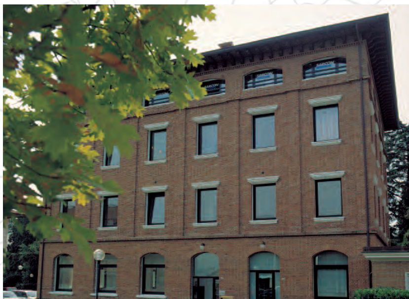
Sede Sarcon / Sarcon Headquarters Thiene (Vi)
